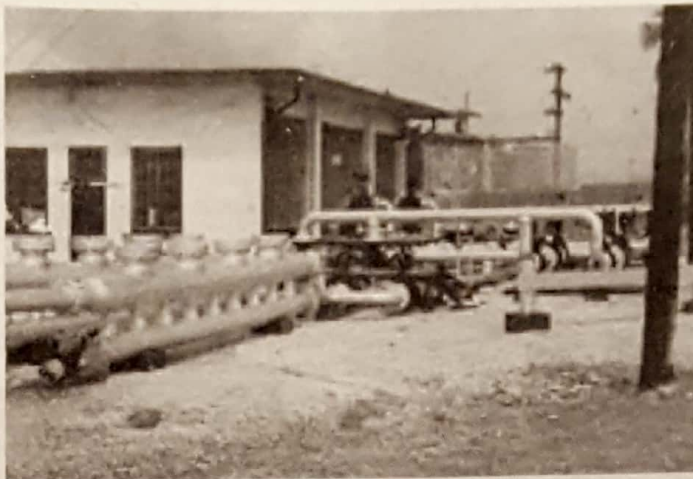
LIFTING THE WEIGHT OFF HIS SHOULDERS: An undated picture of the Cross Island pipeline booster station, where retired Master Sgt. Leroy Foster was assigned. Foster was featured on Florida's WFLA TV, reporting that he has sprayed hundreds of thousands of gallons of Agent Orange while stationed on Guam in the early 1970s. Post file photo
